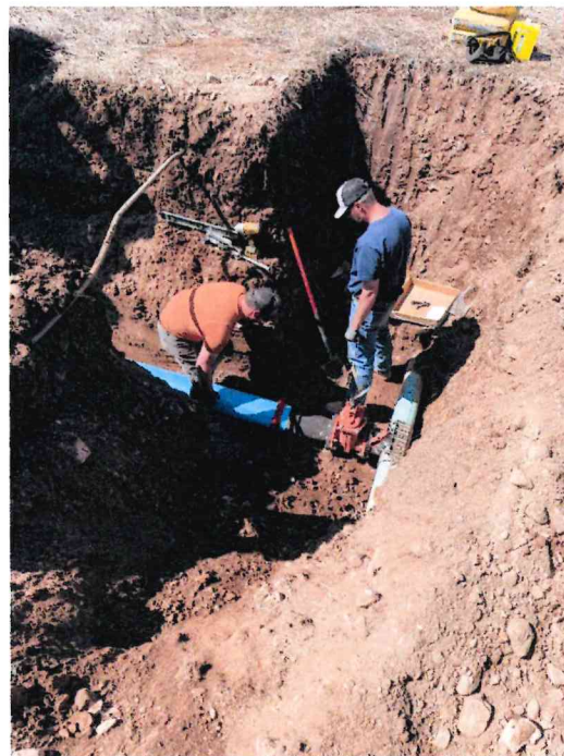
Installing pipe south of water main connection
