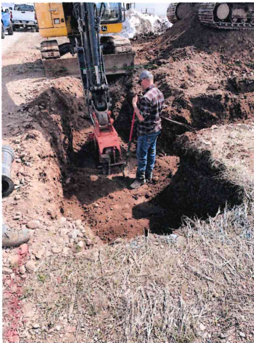
Backfill compaction at water main connection
