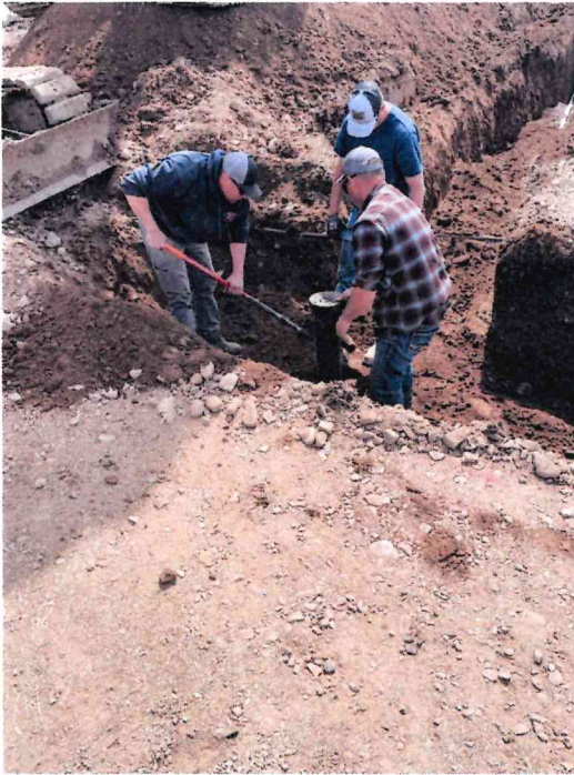
Installing valve riser at water main connection
