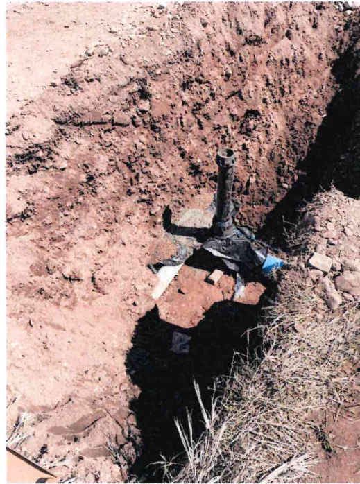
Thrust block at water main connection
