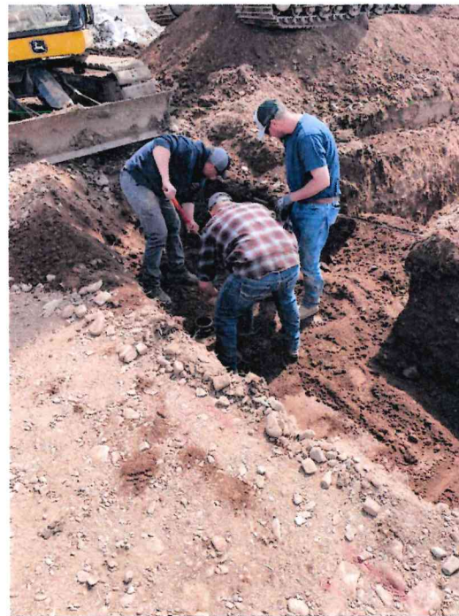
Installing valve riser at water main connection
